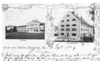
Restauration in Zinneberg
